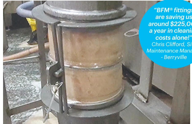
The snap-fit BFM® fitting system with the Tyson clamp
